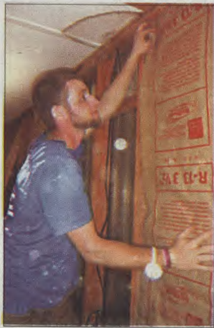
Howard hangs insulation on spring break. Photo by Graham Howard
